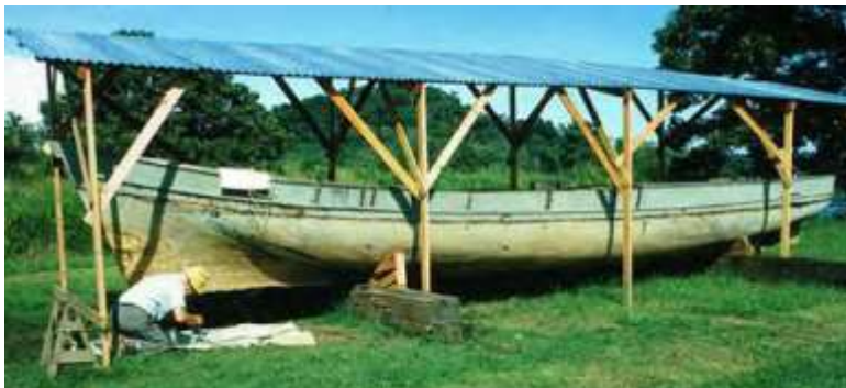
My dad helping with the construction.
