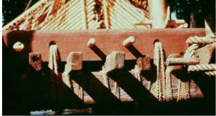
Some of the lashings using coconut fiber rope.
